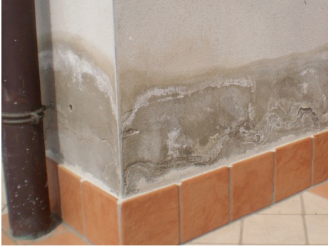
The presence of rising damp on sound plasterwork was easily remedied by removing only the top layers by surface grinding and subsequent application of a Hegea® treatment.
