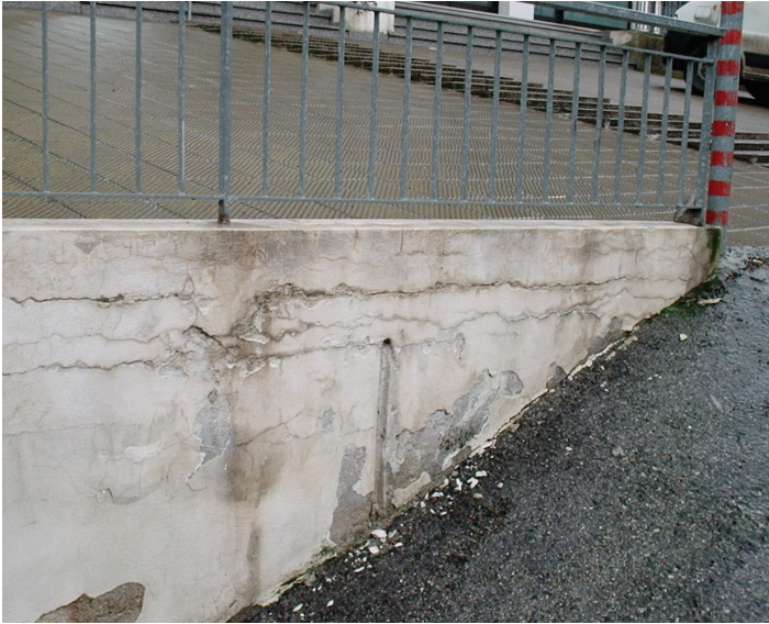
Basement ramp retaining walls with problems of seepage from the soil behind. Treatment with surface sanding and application of negative waterproofing treatment.
