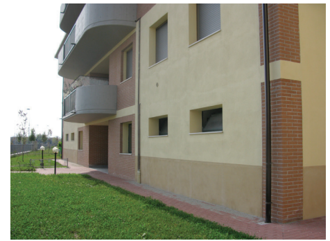
Plaster recently applied but with poor cohesion, affected by capillary rising damp. In order to ensure the proper consistency of the mortars, after removal of the top layers by surface grinding, it was necessary to apply Hegea® Sili Lit deep consolidator. Once cured, apply the Hegea treatment.
