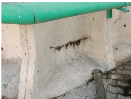
Walls of a sewage water disposal plant, seepages and crumbling originating from the tanks behind. Treatment with surface sanding and application of negative waterproofing treatment.
