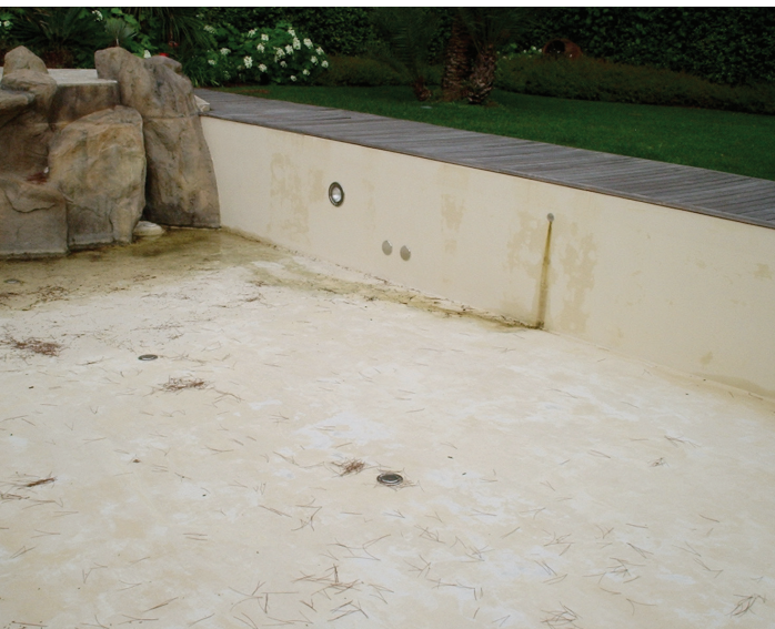
The inside walls of a swimming pool display sections where lifting is taking place and uneven areas. Treatment with surface sanding and application of positive waterproofing treatment.
