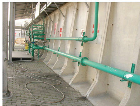
Walls of a sewage water disposal plant, seepages and crumbling originating from the tanks behind. Treatment with surface sanding and application of negative waterproofing treatment.
