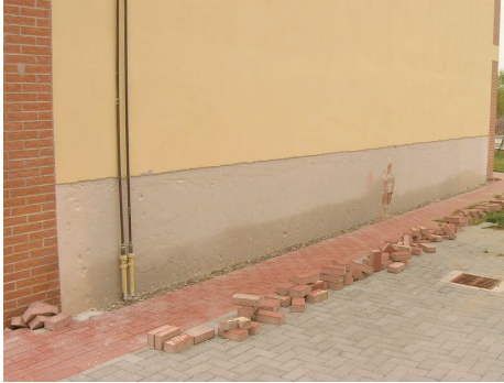
Plaster recently applied but with poor cohesion, affected by capillary rising damp. In order to ensure the proper consistency of the mortars, after removal of the top layers by surface grinding, it was necessary to apply Hegea® Sili Lit deep consolidator. Once cured, apply the Hegea treatment.
