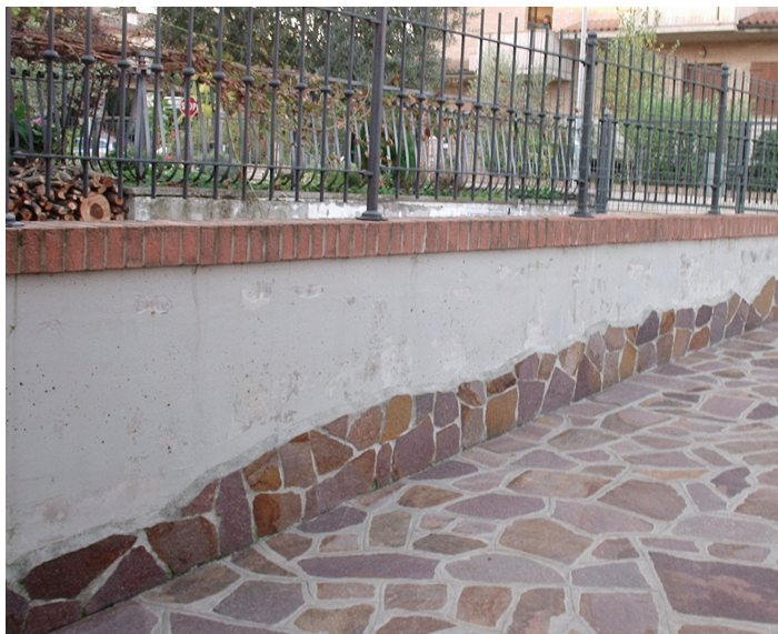
Reinforced concrete retaining walls of basement ramps with problems of seepage from the soil behind. Treatment with surface sanding and application of negative waterproofing treatment.
