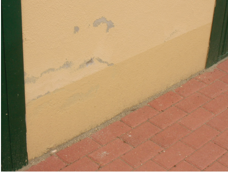
Plaster recently applied but with poor cohesion, affected by capillary rising damp. In order to ensure the proper consistency of the mortars, after removal of the top layers by surface grinding, it was necessary to apply Hegea® Sili Lit deep consolidator. Once cured, apply the Hegea treatment.
