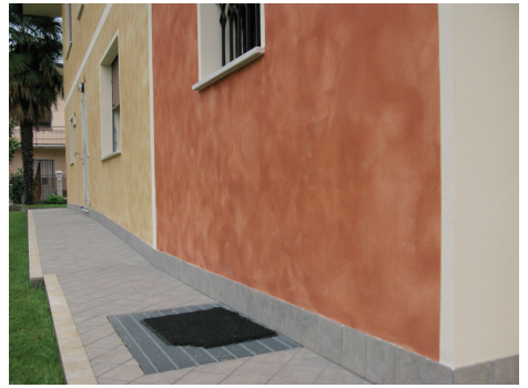
The presence of rising damp on sound plasterwork was easily remedied by removing only the top layers by surface grinding and subsequent application of a Hegea® treatment.
