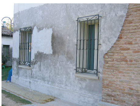
Dwelling with damp problems rising to significant heights, surface sanding, capillary rising damp treatment and interposed mesh.
