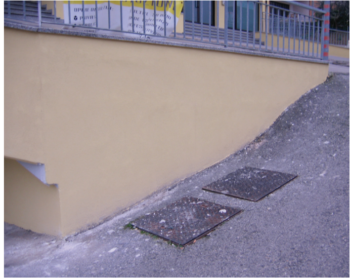
Basement ramp retaining walls with problems of seepage from the soil behind. Treatment with surface sanding and application of negative waterproofing treatment.
