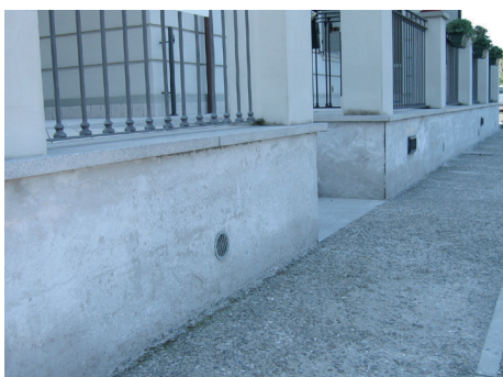
Apartment block with rising damp and crumbling of the perimeter walls, surface sanding and treatment with Hegea products and interposed mesh.
