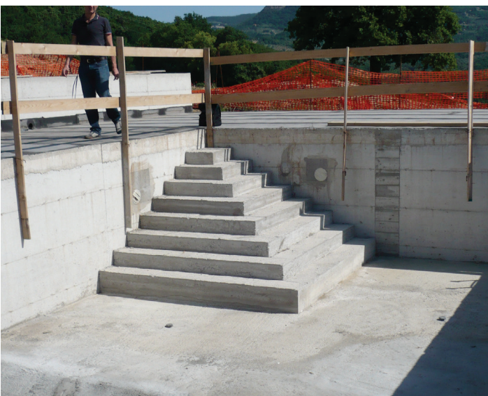
Internal walls of a swimming pool with problems of seepage from the soil behind. Requires water containment treatment and negative waterproofing. Treatment with surface sanding and application of positive waterproofing treatment.
