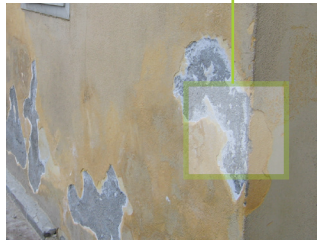
Business property with damp problems at significant heights, surface sanding, capillary rising damp treatment and interposed mesh.
