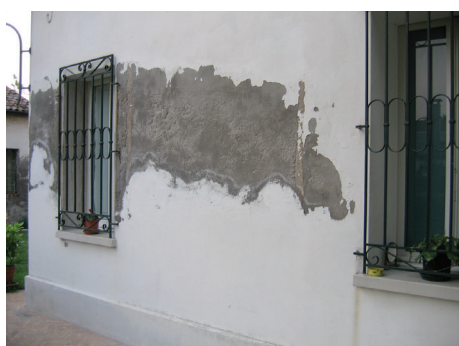
Dwelling with damp problems rising to significant heights, surface sanding, capillary rising damp treatment and interposed mesh.
