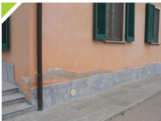
Capillary rising damp, development of efflorescence with lifting of paint and render.
