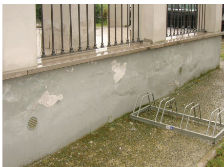
Apartment block with rising damp and crumbling of the perimeter walls, surface sanding and treatment with Hegea products and interposed mesh.
