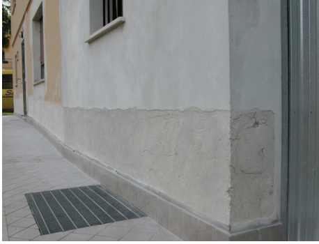
The presence of rising damp on sound plasterwork was easily remedied by removing only the top layers by surface grinding and subsequent application of a Hegea® treatment.
