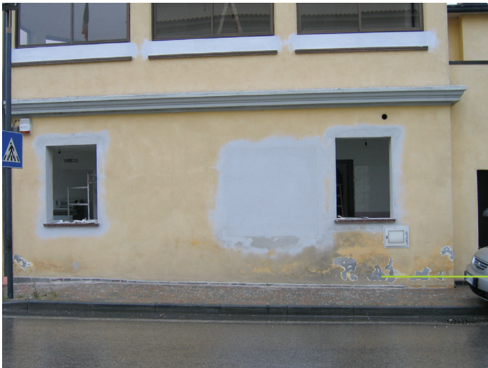
Plaster recently applied but with poor cohesion, affected by capillary rising damp. In order to ensure the proper consistency of the mortars, after removal of the top layers by surface grinding, it was necessary to apply Hegea® Sili Lit deep consolidator. Once cured, apply the Hegea treatment.
