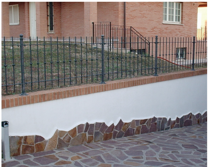
Reinforced concrete retaining walls of basement ramps with problems of seepage from the soil behind. Treatment with surface sanding and application of negative waterproofing treatment.
