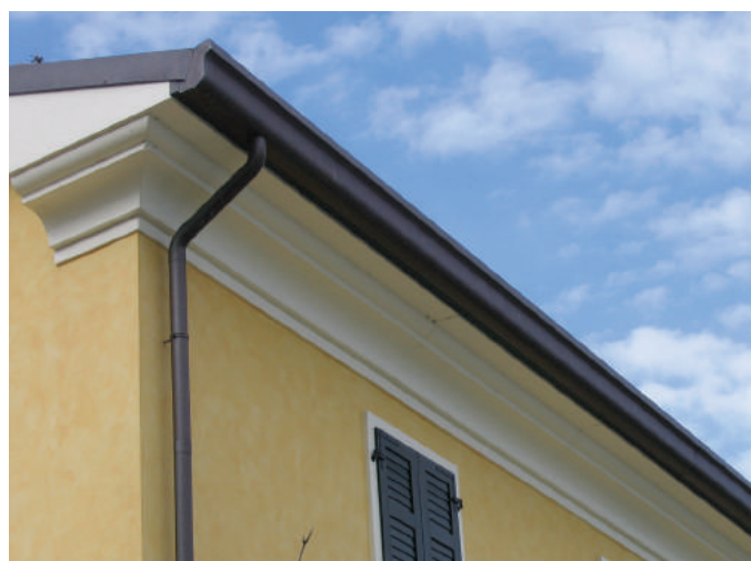
SG.H.4040: Under-eave cornice Height 400 mm Depth 400 mm Length 1000 mm
