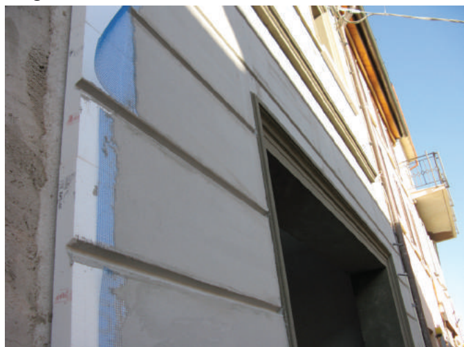
FC.H.4380: Cladding strip treatment only on the joint Height 430 mm Depth 80 mm Length 1000 mm
